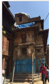
Walking through buildings propped with 4x4s!
